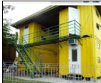
In response to the need to get our boys' dormitories and library built soon, we are going to have them constructed out of shipping containers. For much less cost than building a cement block building, they will be insulated, electrified and re-roofed. Each container is 8'x40' and can be arranged in a number of ways, including stacked (as in this example photo) and two joined together. We will be able to put the rental monies of \$1,000 per month
